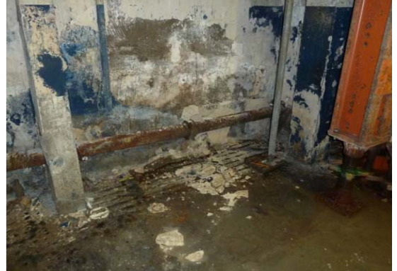
Water damage and condensation issues to the basement. (Source: Curteis, Preliminary assessment of the environmental conditions associated with the conservation and redevelopment of the lion chambers, Glasgow. June 2015.
