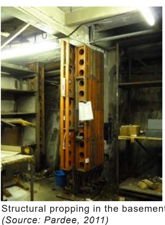
Structural propping in the basement (Source: Pardee, 2011)
