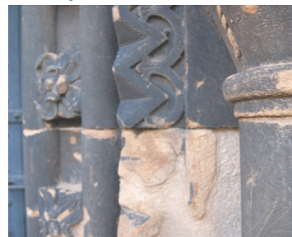
Loss of detail in areas where the black crust has come away from the stone.
