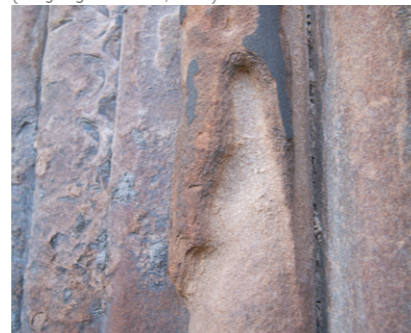
Visible migration of iron oxide and mineral cements to the outside face of the stone, leaving a powdery inner stone lacking cohesion.
