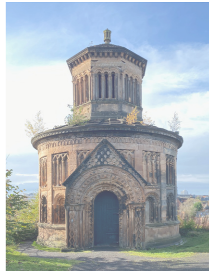
Monteith Mausoleum entrance, facing south-east (image by MacKenzie, 2020)
