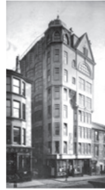
Lion Chambers, 1910 (RCAHMS) The second fully reinforced concrete framed building in Glasgow.
