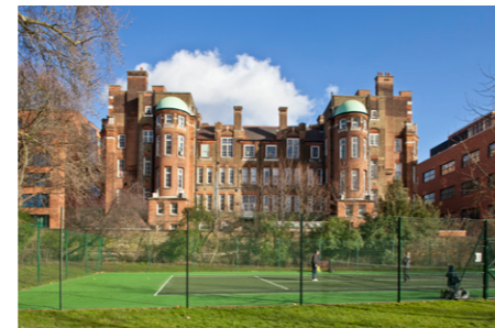
Rear elevation of the King's Library
